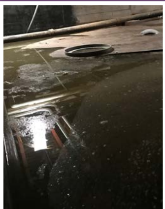
Above, flooding in the basement at Union Springs MS/HS. Pipes are clogged, compressed, corroded, or broken, and seemingly a source of continuous repair.
