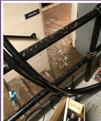
Above, flooding in the basement at Union Springs MS/HS. Pipes are clogged, compressed, corroded, or broken, and seemingly a source of continuous repair.
